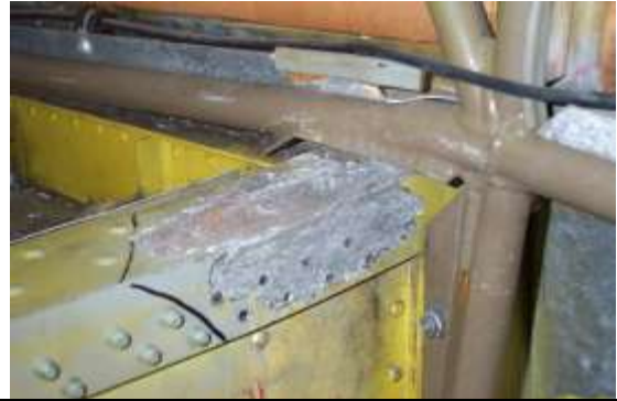
Main Spar- corrosion found under the rear seat upholstery
